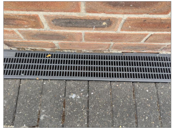
Photo - 16 Extend the soakaway grid around all the walls
