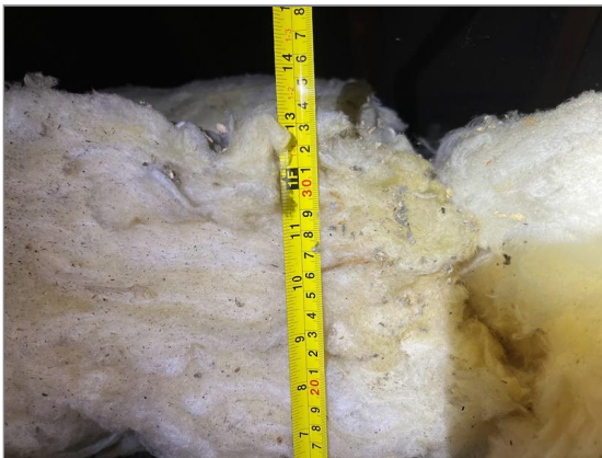
Photo - 29 Loft insulation - approx 330mm.
