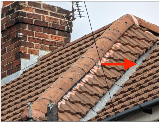
Photo - 9 Valley gutters ok
