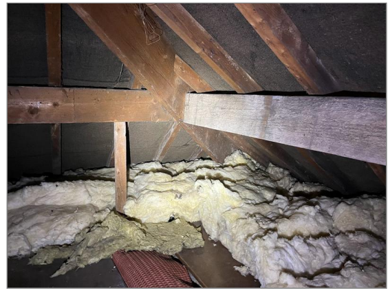
Photo - 28 Roof structure.
