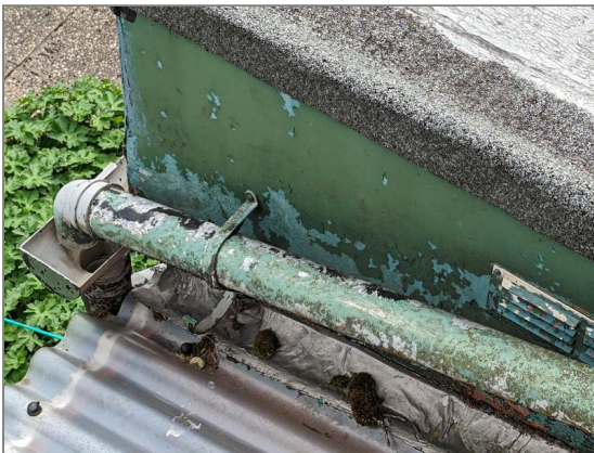
Photo - 12 Dated rainwater goods
