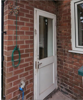
Photo - 20 Timber rear door - dated.
