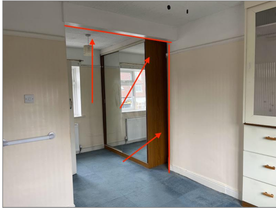
Photo - 32 Internall wall removed.
