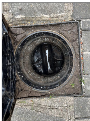
Photo - 47 Mains drainage - clear.
