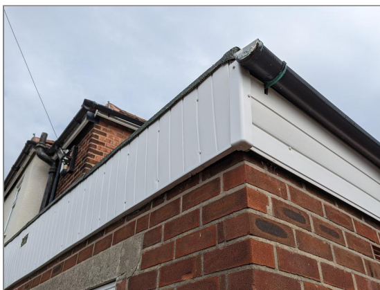
Photo - 23 Plastic roof joinery satisfactory
