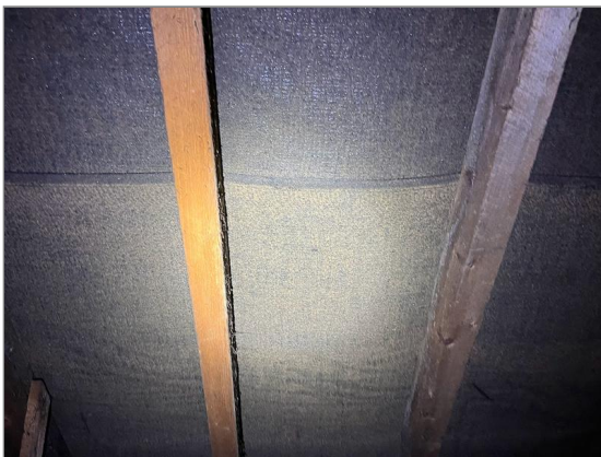
Photo - 7 Secondary waterproof layer (roofing felt).
