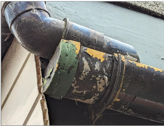
Photo - 10 Dated rainwater goods
