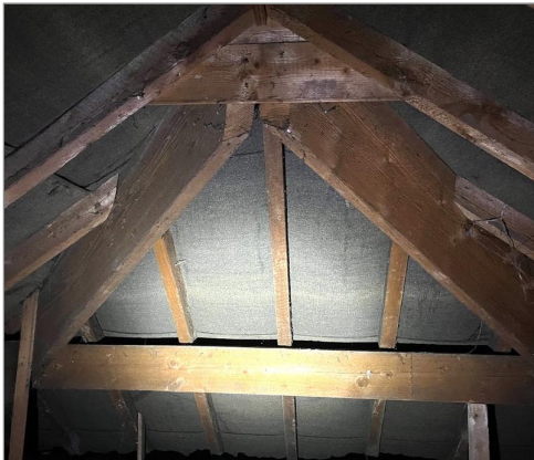
Photo - 25 Roof structure.
