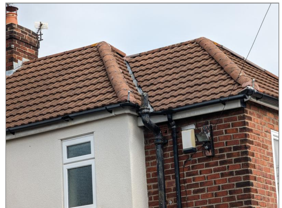
Photo - 8 Replacement roof coverings satisfactory
