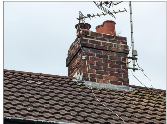
Photo - 4 Rear face of shared stack
