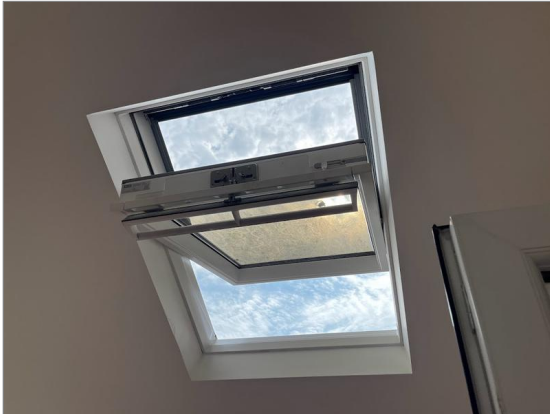
Photo - 18 Velux rooflights - satisfactory.
