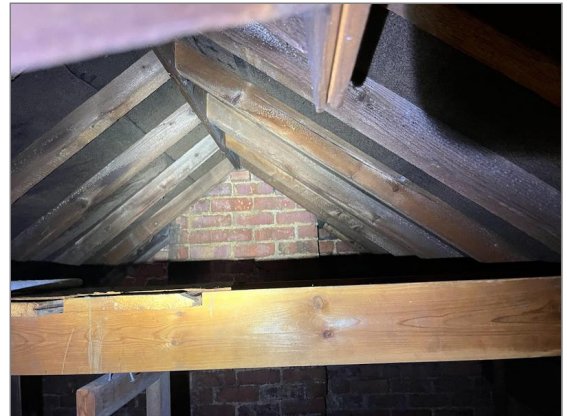
Photo - 26 Roof structure and party wall.
