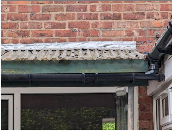
Photo - 50 Dated canopy at rear of house
