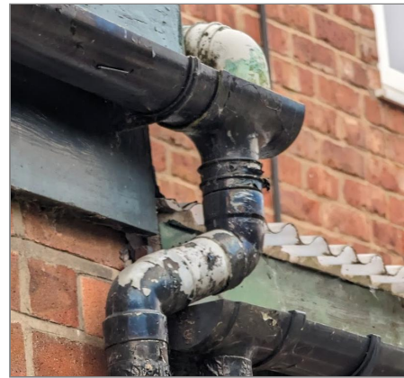
Photo - 11 Dated rainwater goods
