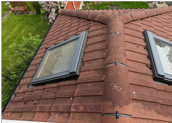
Photo - 21 Ensure adequate support for the concrete tile roof
